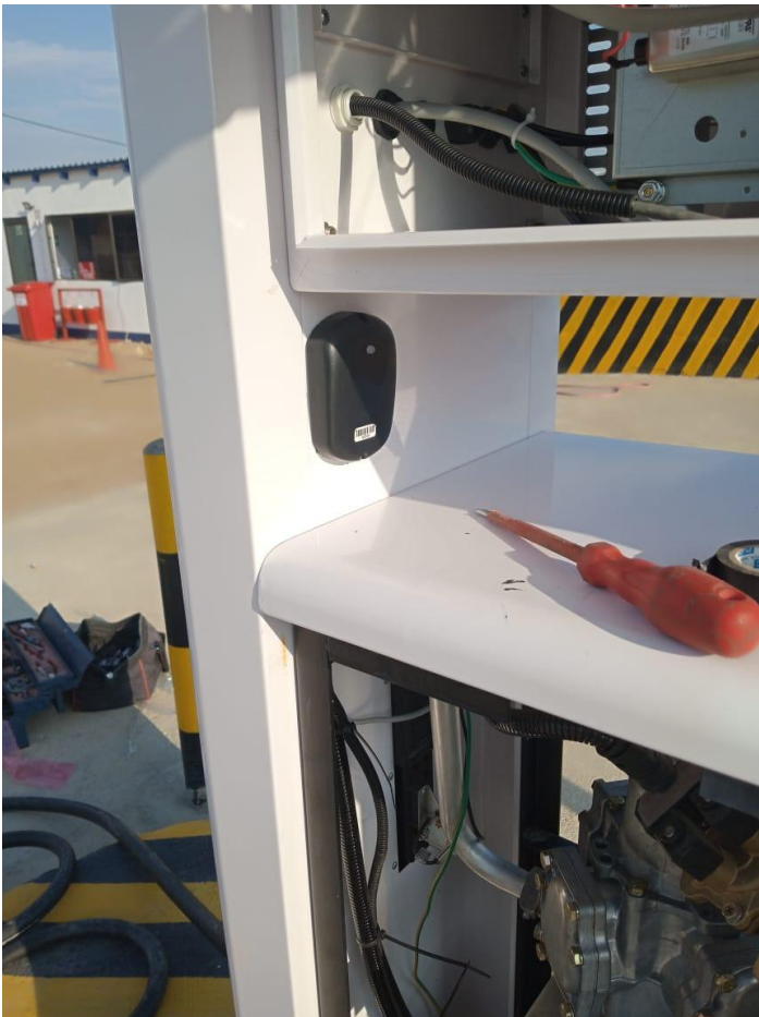
Example of reader installation on fuel dispensers
